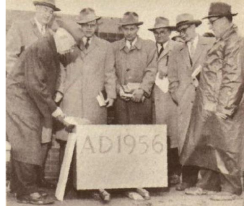
From left to right are Dr. I.E. Bradfield, Synod Executive; Mr. Herbert Moore, Moderator of Milwaukee Presbytery; Mr. Ferd Shoenbaum, Jr., General Chairman of the Building Program; Mr. Werner Blom, Chairman of the Plans and Construction Committee; The Rev. John Dzuro, Pastor of Greenfield Ave. Presbyterian Church and former pastor of Forest Park Church; Dr. A. Gladstone Finnie, Chairman of Milwaukee Presbytery's Committee on National Missions; and the Rev Garth Gee, pastor.
